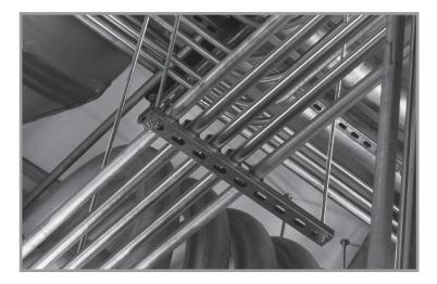
12 clamps are needed for the installation of 12 conduits of 1"
