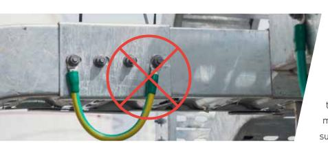
Compliance with the standard ensures that the system has electrical continuity, and therefore, it is not necessary to use additional connections between the parts to ensure a correct bonding between them when installed according to the manufacturer's instructions and with suitable accessories.
